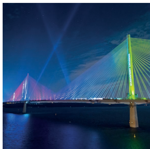
CXL Type A and Type C Couplers, Queensferry Crossing, UK (Photo courtesy of Transport Scotland)
