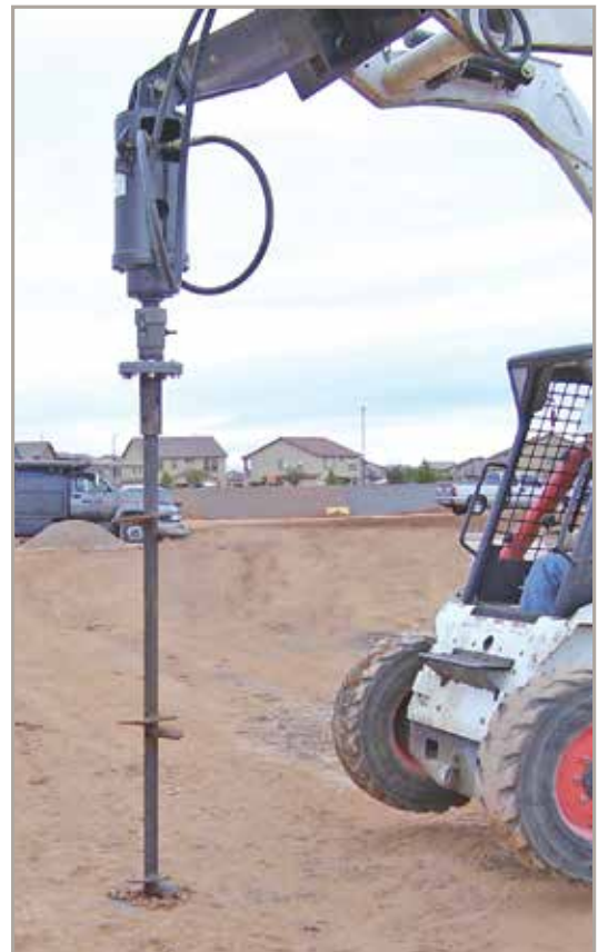
Typical MB Brace Badger Installation
